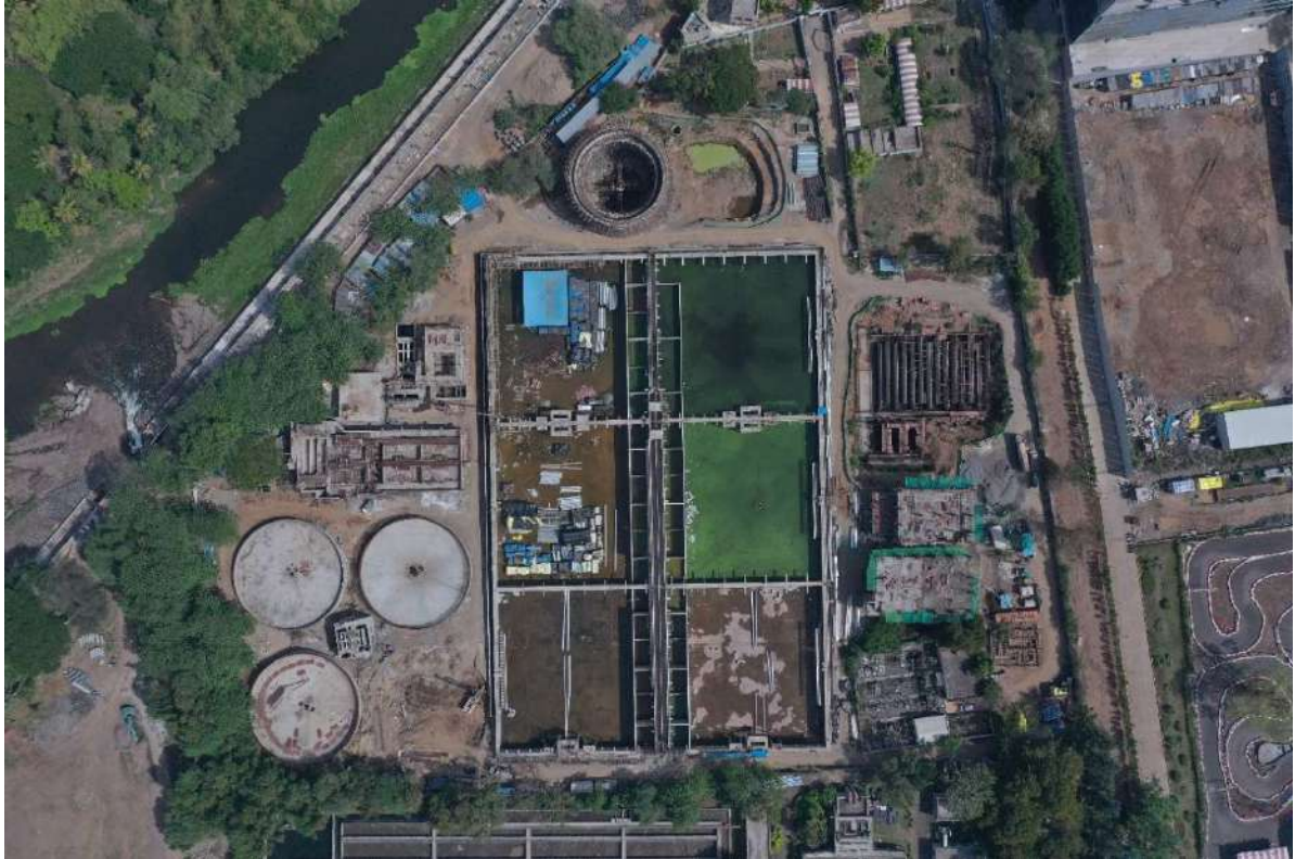
( Dr. Naidu Sewage Treatment Plant – ૧૨૭ MLD )
