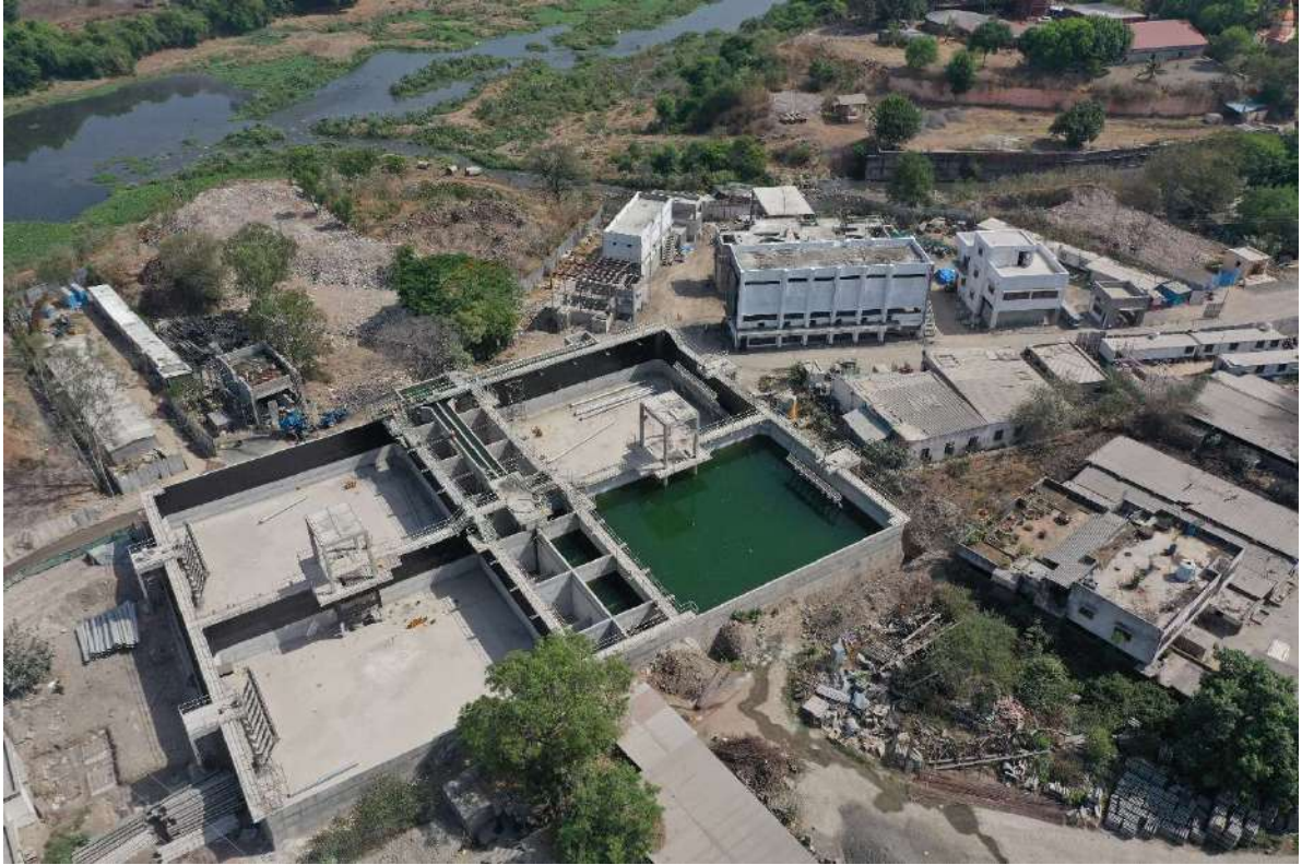
( Vadgaon Sewage Treatment Plant – २६ MLD )
