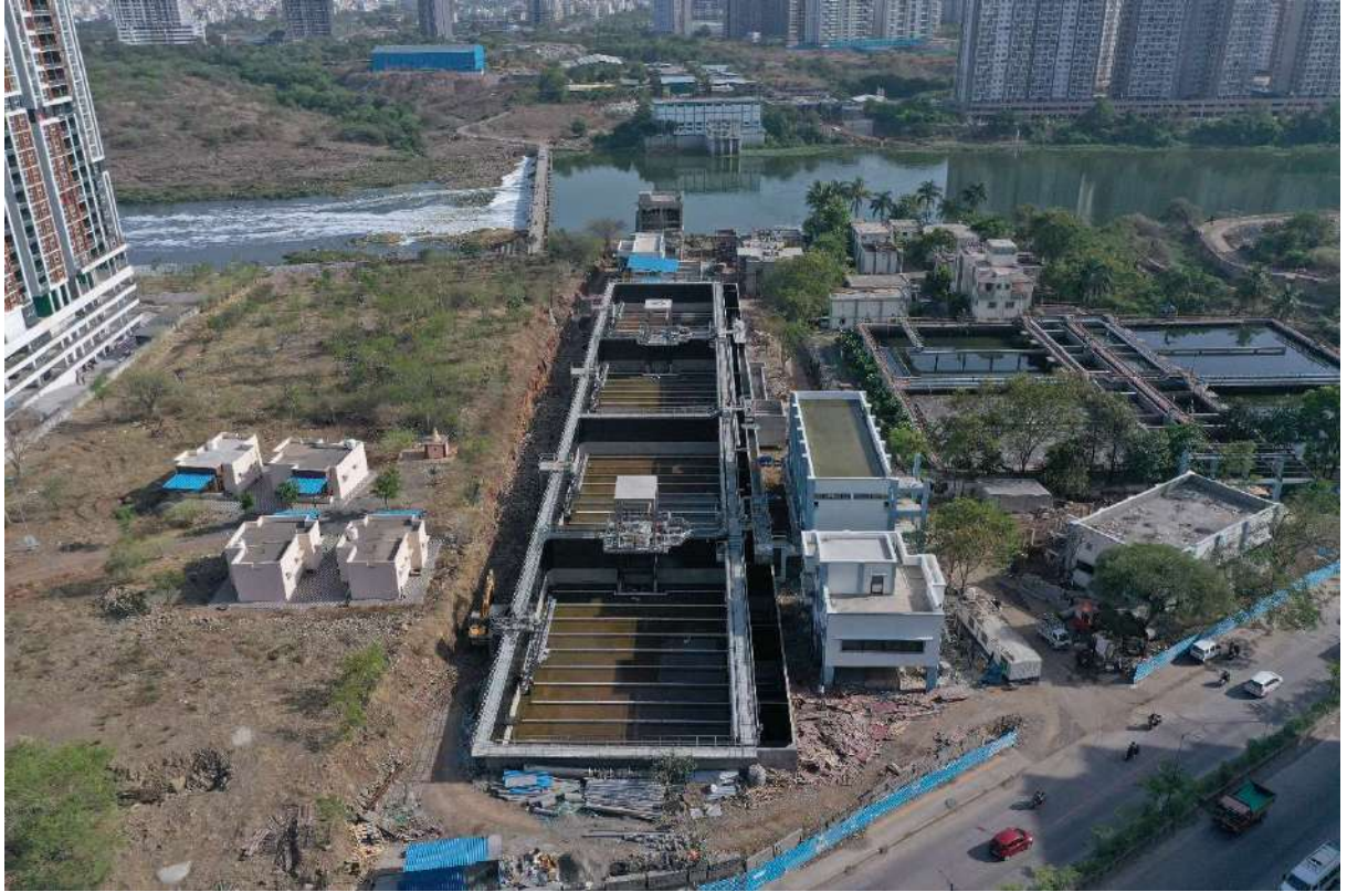
( Kharadi Sewage Treatment Plant - ३० MLD )
