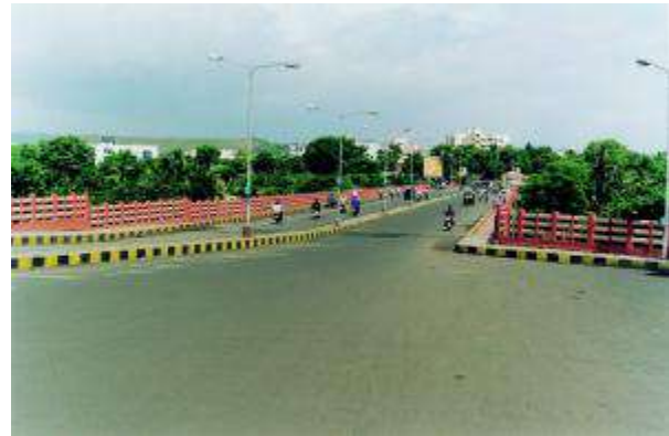
Shri. Chhatrapati Rajaram Bridge: Waiting for connection from river side road
